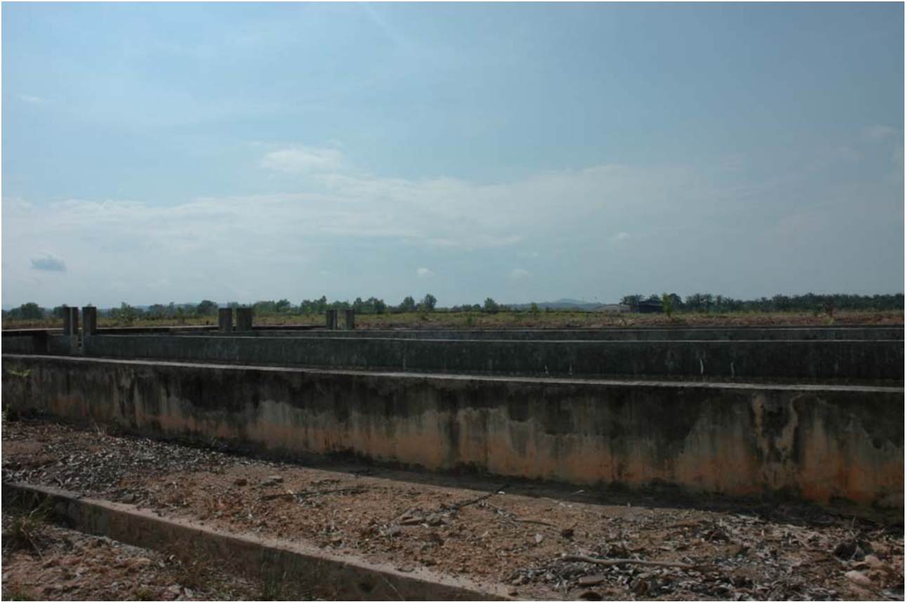
Waste Treatment Plant of PFA NS (污水管理设备)
